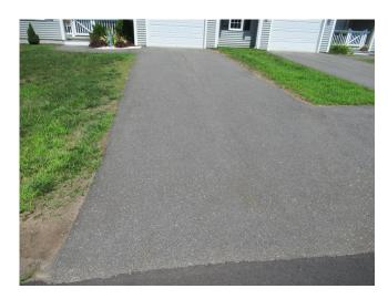
Component budget covers rebuild of asphalt driveways. Asphalt was in good condition at site visit. Component listed separately from roads due to longer driveway typical useful life and higher cost per sq. ft. for rebuild vs. overlay. Driveway area equates to 5240 sq. yds.
