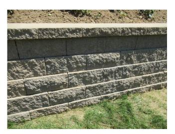
Component budget covers landscape block retaining walls adjacent to building 33. Walls were in good condition at site inspection.
