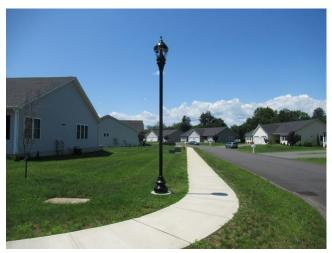
Component budget covers site post lights. Lighting was in good condition at site visit. Cost assumes that post light wiring and concrete bases can be reused. Fixture quality and size will affect cost significantly.
