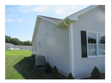
Component budget covers replacement of vinyl siding over 2 years. Siding is comprised of double 4" vinyl clapboard in standard colors. Siding has average trim details and was in good condition at site visit.
