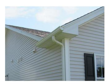
Component budget covers replacement of aluminum 5" gutters and 2"x3" downspouts on units. Frequently, gutter replacement coincides with roof replacement. However, with longer life roof shingles, replacement may be needed sooner. Gutters were in good condition at site visit. Remaining life should be updated in future reserve study updates.
