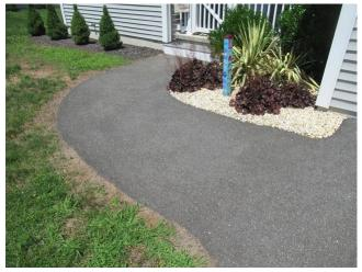
Component budget covers asphalt walkways to unit front doors. Walkways were in good condition at site visit. Lower unit cost used in anticipation of replacement of walkways in conjunction with driveways.
