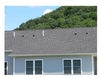
Component budget covers removal & replacement of unit asphalt architectural shingle roofs over two years. No roof issues were reported. Per client, roof shingles have 50 year warranty. Useful life set at 40 years for unproven longer life shingles.
