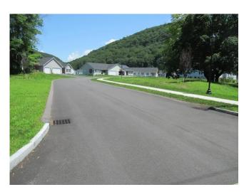
Component budget covers asphalt driveway and walkway maintenance. Asphalt is in good condition. As infrastructure ages, allowance should be adjusted in future reserve study updates.
